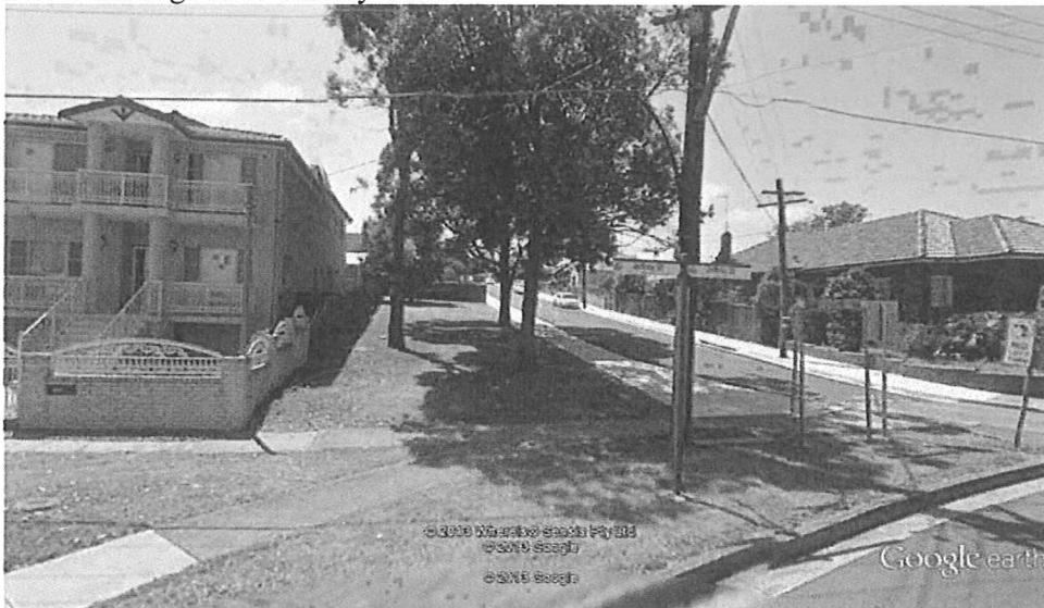
Street frontage at 49 Jeffrey Street
