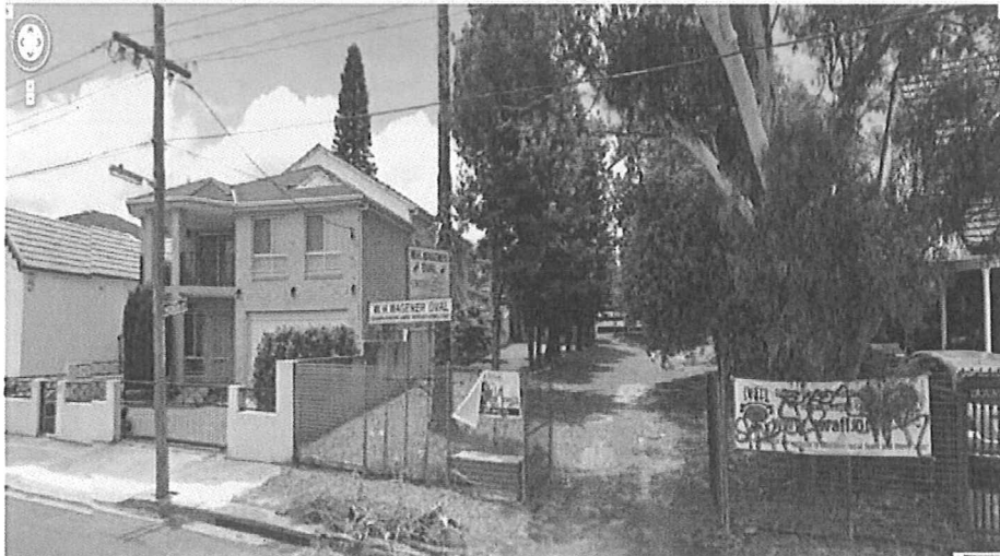
Street frontage at 2 Whitfield Avenue
